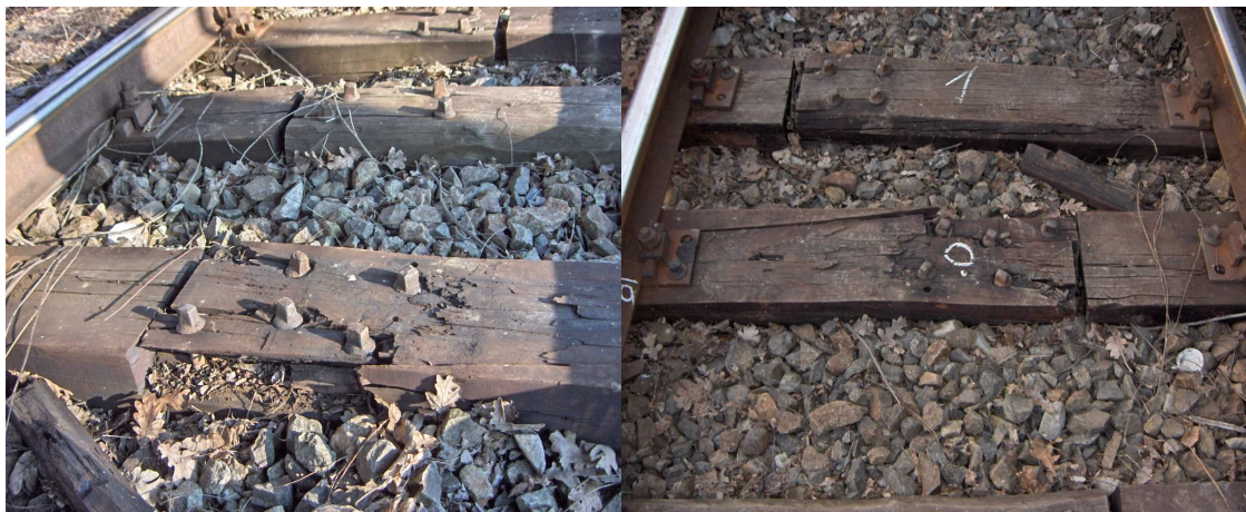
Photo 6: breaking of the joined sleeper “0”
