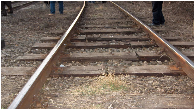
Photo 5: line in the derailment area and joining the sleepers
